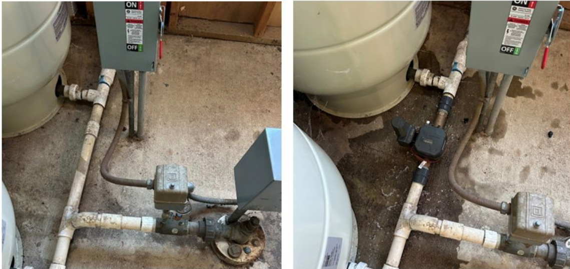
Figure 2. Photographs of a Typical Flow Meter Installation (Before and After)
